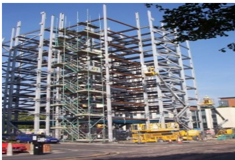
Fig 3.4 showing a Vertical bracing in a multi-Storey building
